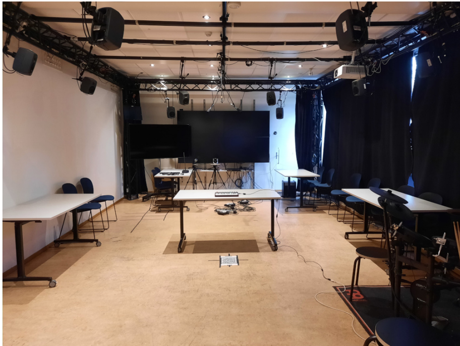
Figure 4.16: The performance area in the MCT Portal . The loudspeakers array for the spatial audio system is placed under the rooftop as well as the cameras for the motion capture system (no much noticeable). Moreover, it can be found in the center a table with the MIDI controller and several other furniture that can be used for placing the spatial positioner .
