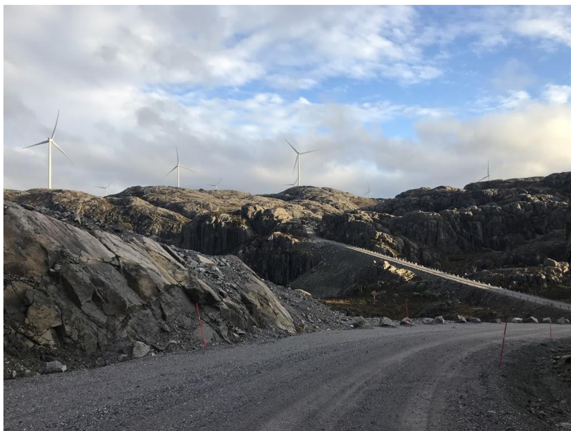
Figure 2: Example of the dirt roads that connect the turbines. Road cuts is also visible in this photo. Photo: Aggie Handberg
