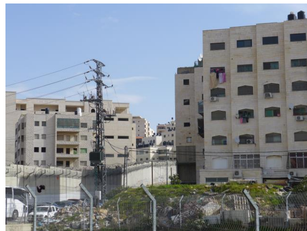
Security barrier, deemed illegal by ICC, going through a Palestinian neighbourhood in East Jerusalem. (Photo by author)
