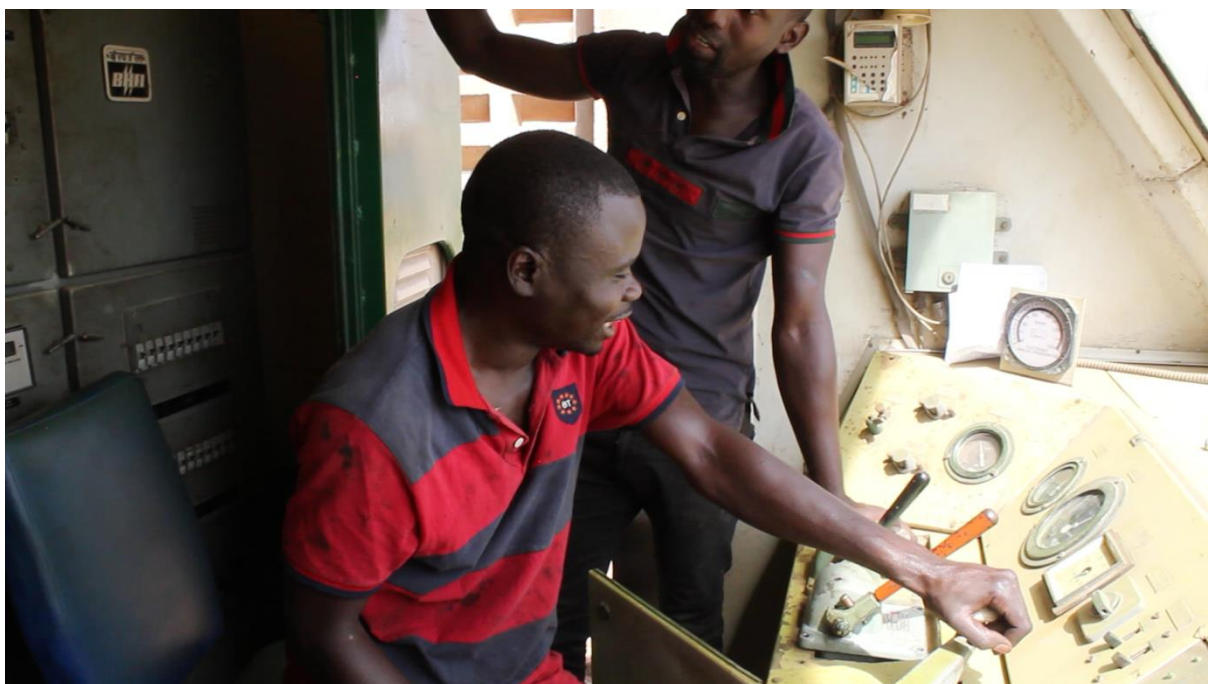
Fig. 1 and 2. Repair works in the depot of Rufisque 2
