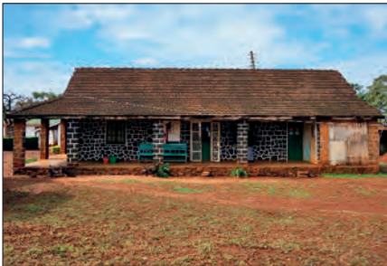
Figure 2: Original building of Kibong'oto Hospital. It was demolished in 2018. (Photo: Christoph Gradmann)
