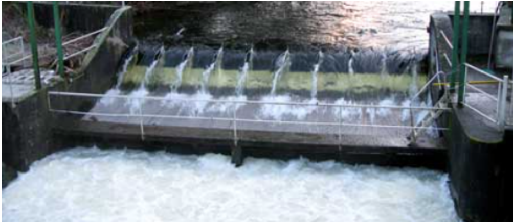
Picture 2.1: The Wolf trap located at the bottom part of Imsa (Photo: Knut Bergersen, NINA).
