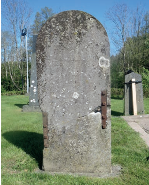
85. The back of a narrow, rounded limestone gravestone from the 1880s repaired with iron in Långelanda. The limestone was broken in previous times. Photo Anders Gustavsson.
