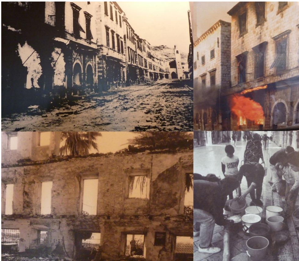
Figure 12. War damage on the walled city of Dubrovnik and surroundings. Photograph above left: Dubrovnik's main street, Stradun (Placa) , after shelling, above right: house in the walled centre on fire, below left: a 'skeleton' of a house left after torching and shelling, and below right: locals collecting water brought to the walled centre by outside volunteers during the Dubrovnik siege. Photographs published with permission from the Dubrovnik War Museum.
