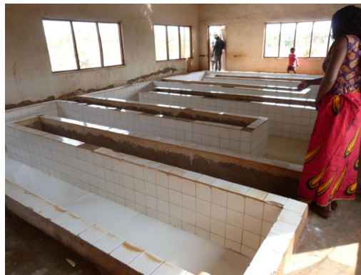
Picture 10. Starch settling tanks
