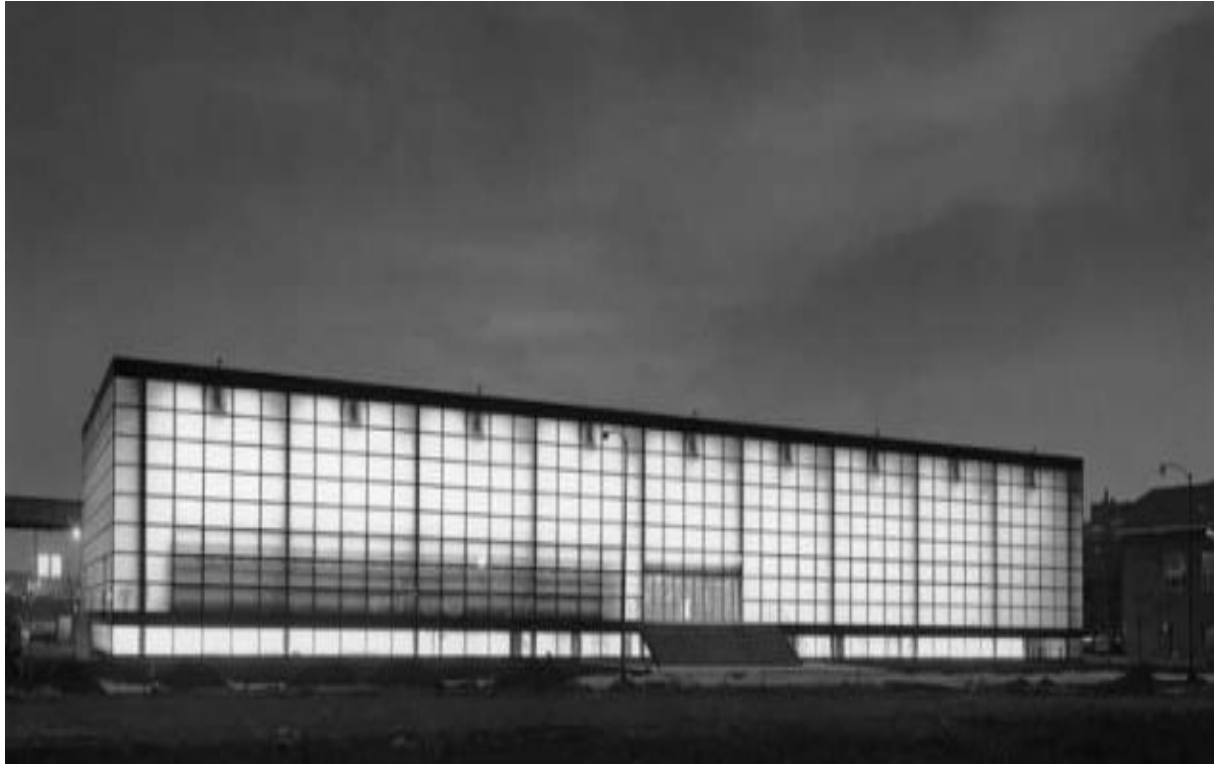
III. 48. Mies van der Rohe: Mineral and Metals Research Building (1943), Illinois Institute of Technology.
