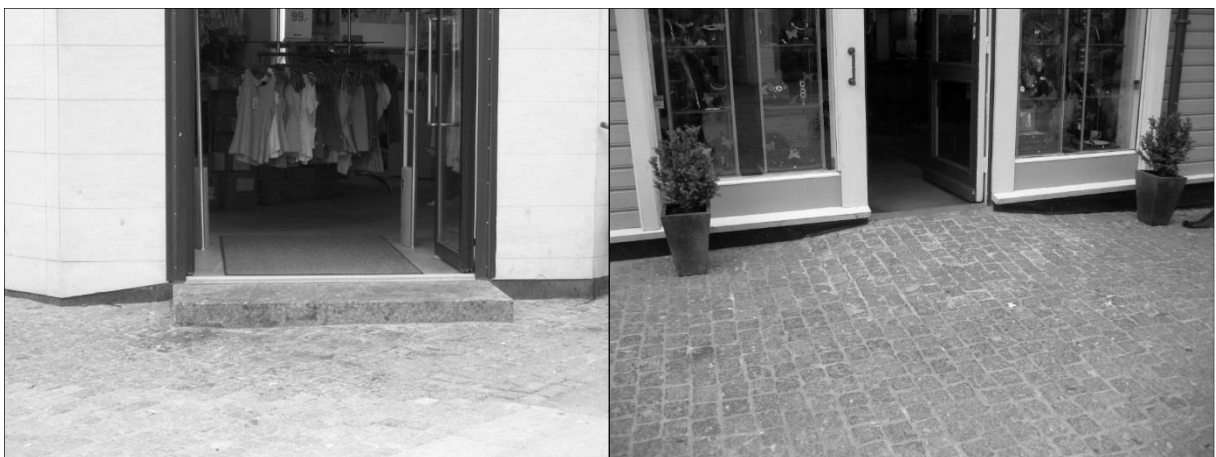
Figure 4 : Entrances with and without physical barriers. Photo by Tone Moseid, reproduced with permission
