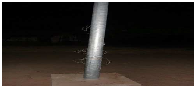
Plate 8: The street light with a protection wire
