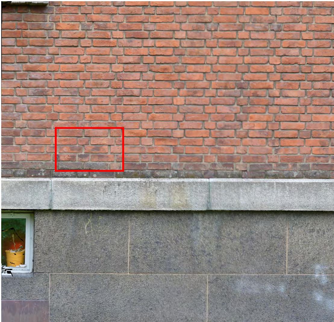
FIGURE 3.7: Resulting ortho-photo from the test for speed vs. quality. The section highlighted in red was used for point cloud analysis.
