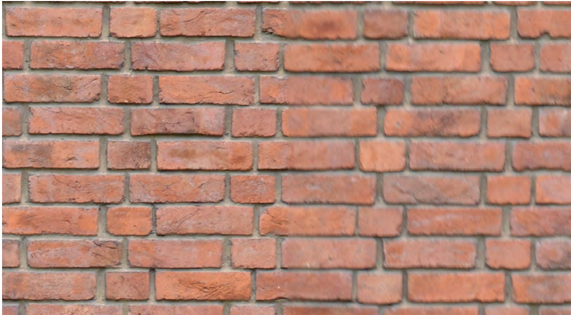
FIGURE 3.4: This figure shows an ortho-photo composed of a mosaic of the original images. The image used for the right hand portion was out of focus. A total of 4 images were used in the processing.
