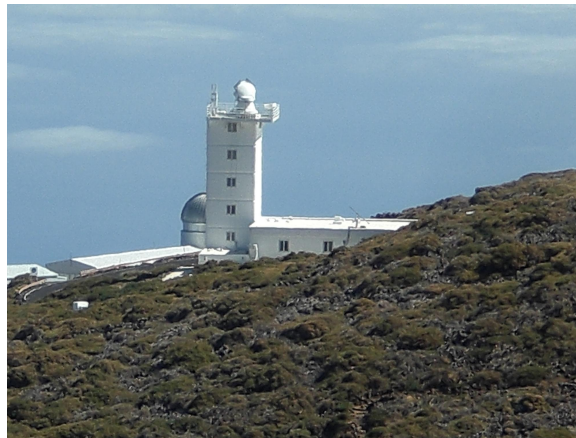
Figure 2.1: The Swedish 1-m Solar Telescope at 2400 m, within the Observatorio del Roque de los Muchachos, at La Palma. On top of the 15 m high vacuum tower, the turret with the 1-m lens tracks the Sun throughout the day. (The Mercator Telescope is seen in the background.) (Photo: Elisabeth Jordahl)
