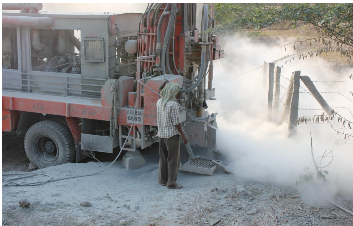
The boring of a bore-well near Aurepalle, Andhra Pradesh, 2013.
