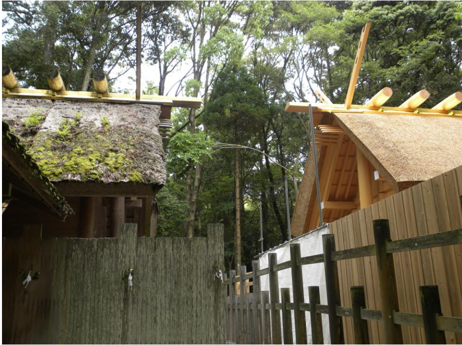
Figure 19: Before the shikinen sengū: an old shrine building next to a newly-built one
