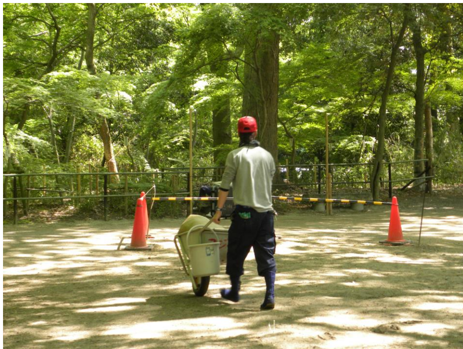
Figure 5: Forest maintenance work at Tadasu no Mori
