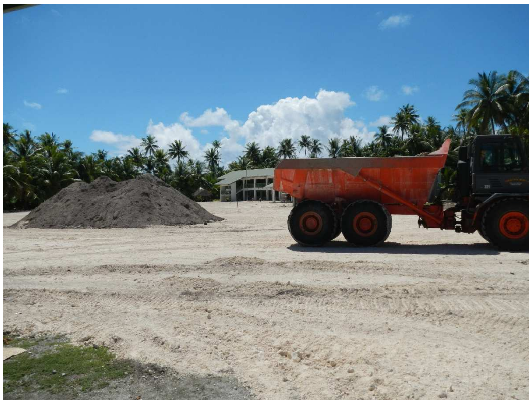
2.6 The area after the removal of the bush
