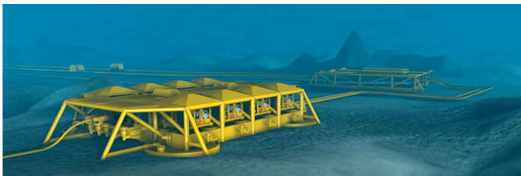
Fig 53 Artists impression of Sub sea well template containing wellhead control equipment, in the background start of 80 km double multiphase transport pipelines to land processing plant ©Hydro/ Ormen Lange project homepage
