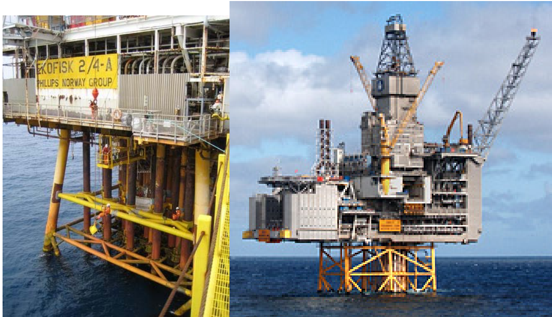
Fig 20 Ekofisk steel jacket platform © unknown Fig 21 Oseberg Sør, a 1990s Steel platform © Hydro
