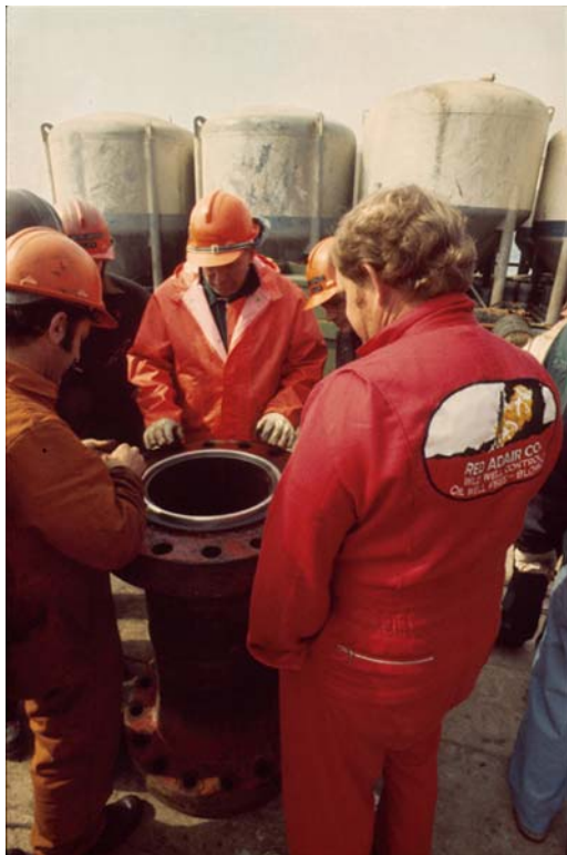
Fig 46 The wellhead on the Bravo platform after recovery © Norsk Olje museum
