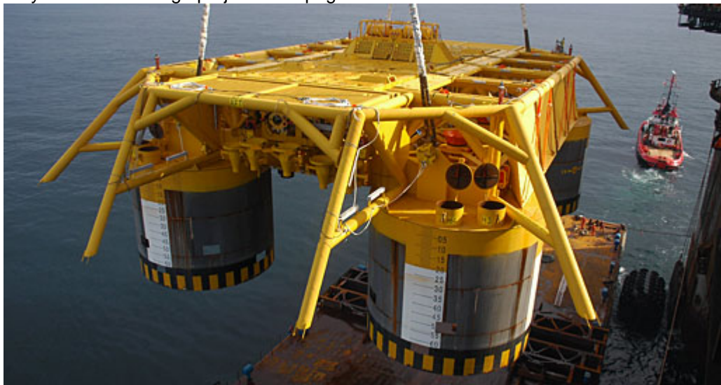
Fig 52 Dimensions of the sub-sea well template for four wells with control equipment ©Hydro/ Ormen Lange project homepage
