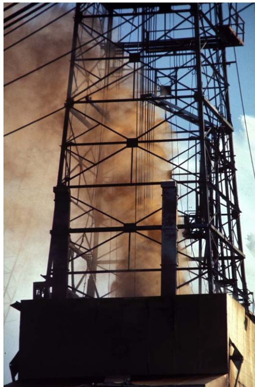
Fig47 Oil blowing out through the derrick of the Ekofisk Bravo platform © Norsk Olje museum
