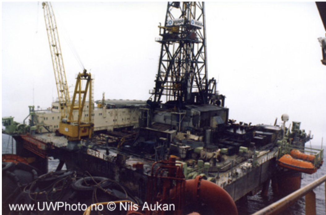
Fig 49 West Vanguard after the blowout – fire/explosion damage to the main deck and the list of the rig is clearly visible ©Nils Aukan/ANS agency
