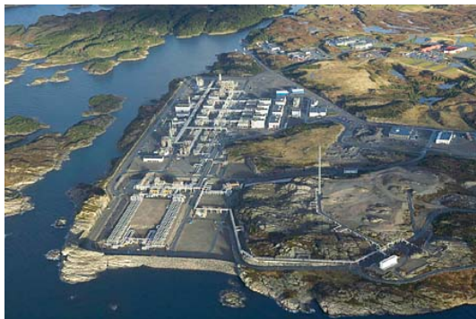
Fig 35 Gas processing plant at Kollsnes © PSA
