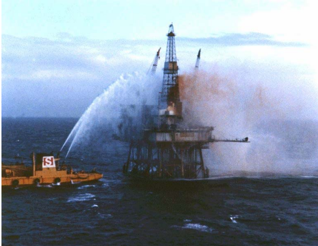
Fig 45 Ekofisk Bravo platform blowout of oil - to the left a supply vessel spraying water to avoid ignition of the oil © Norsk Olje museum
