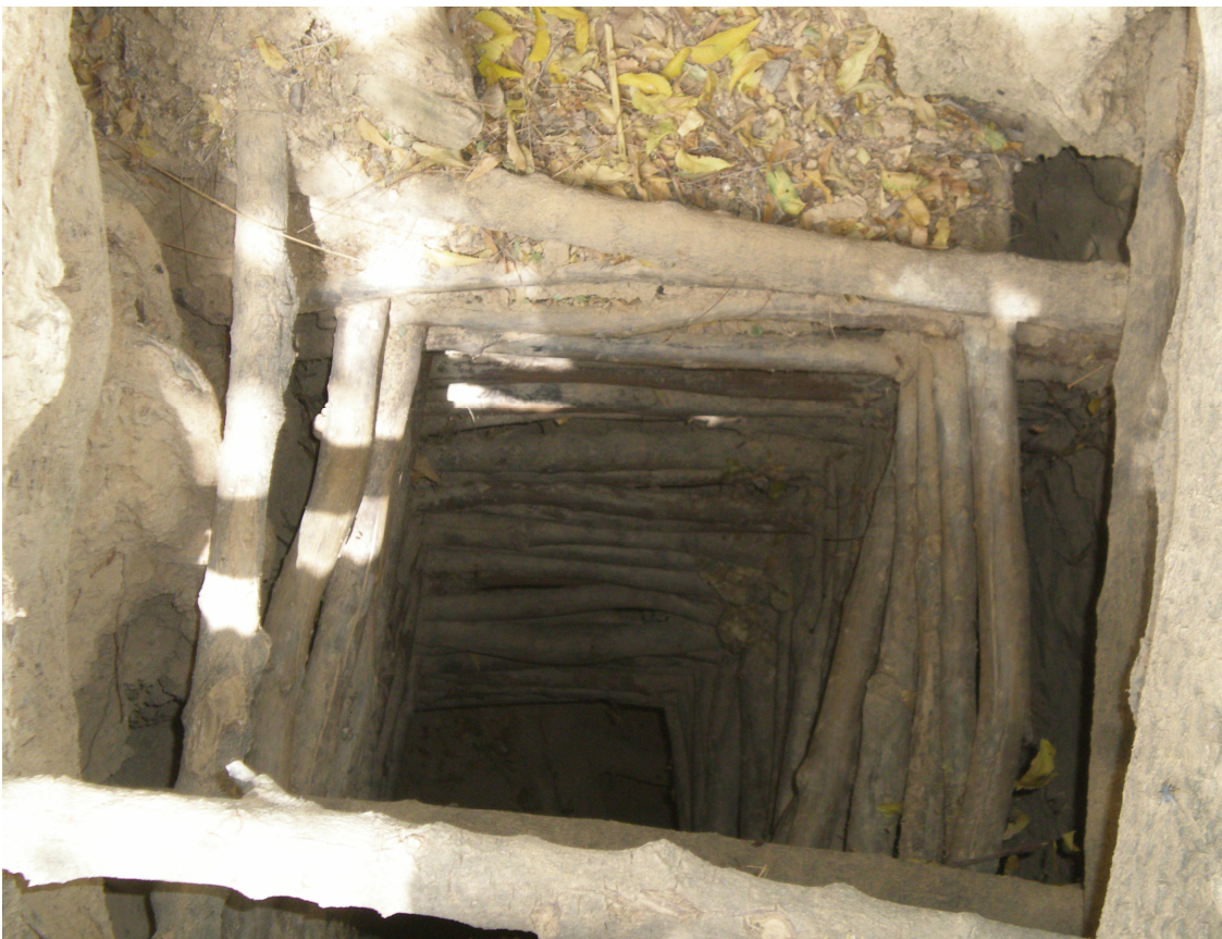
Figure 4.5: A wooden structure used to prevent the pit from carving in.
