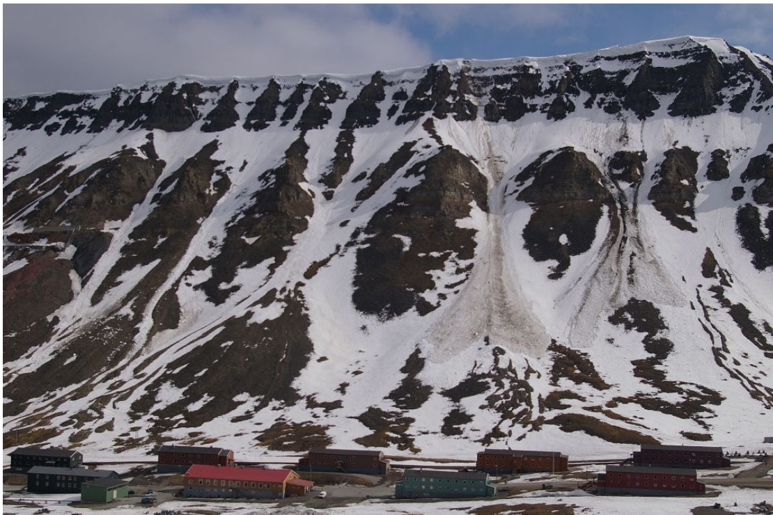
Figure 14 Automatic time lapse photograph of the 'Sverdrupbyen' camera across the valley Longyeardalen from 2 June 2010. Large failures are visible in the gullies 'Wrong Step', 'Willy Sagnol' as well as remnants in 'Triple Y'. The houses of Nybyen are in the lower part of the photograph and the mine to the very left.
