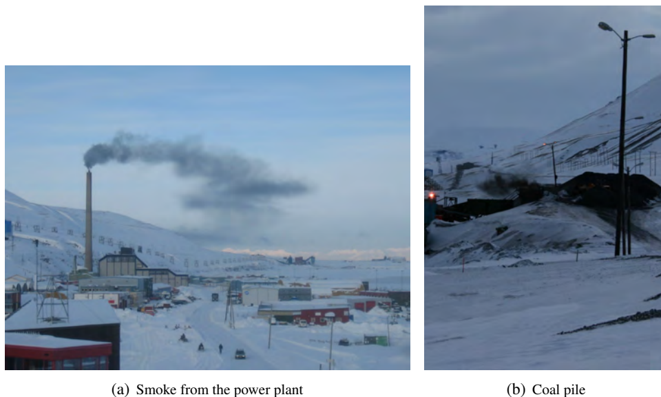
Figure 2.4: (a): Black smoke from the coal power plant in Longyearbyen on the 30th of March 2009. During that particular episode, the exhaust was not cleansed. (b): Airborne coal dust seen as black smoke at the coal processing plant nearby Longyearbyen on the 19th of February 2008. Photo by Åsmund Aamaas.
