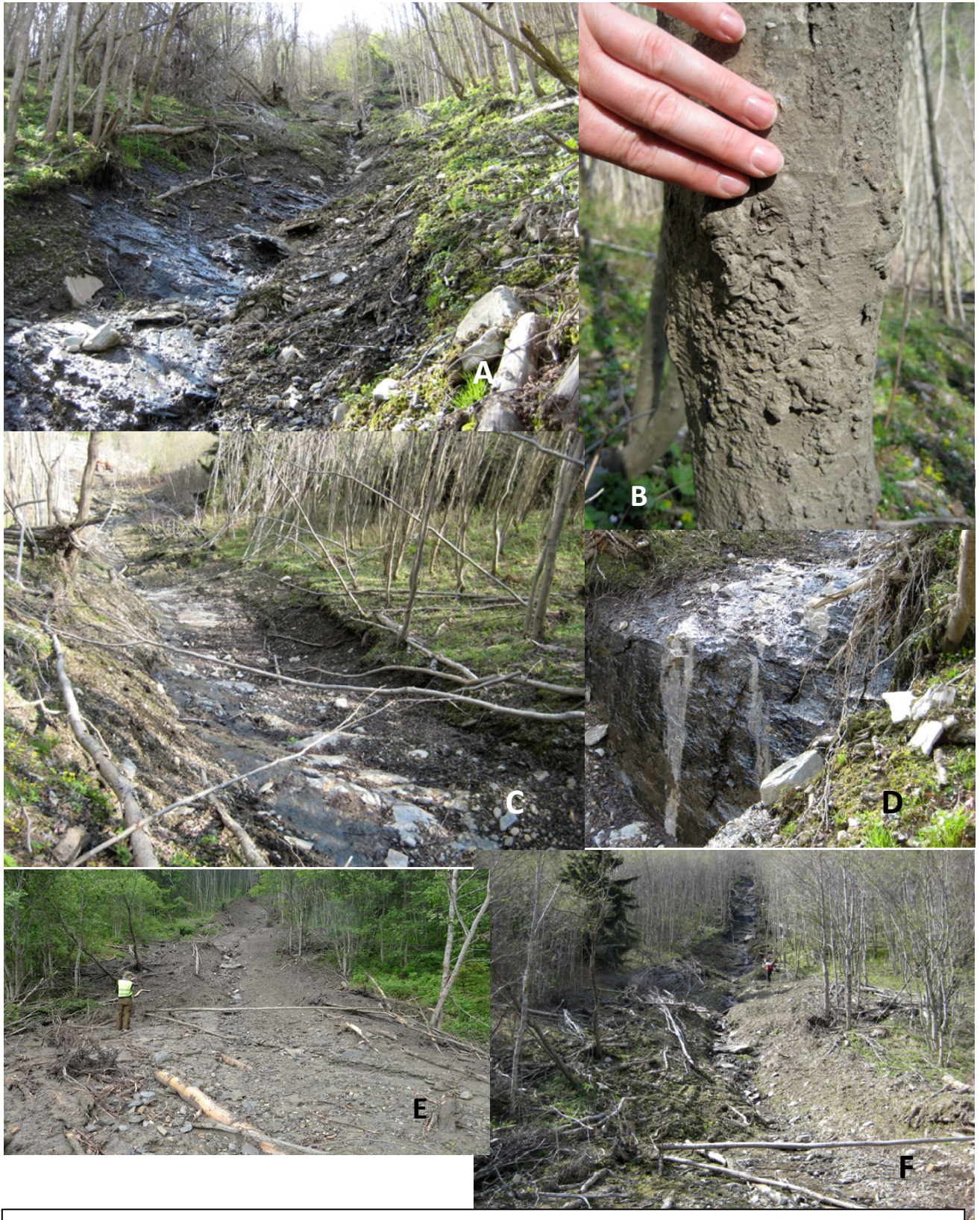
Figure 3.21 Section two of Landslide two. A , Upper track of landslide, looking west. B , 1 cm thick mudmarks on trees close to landslide track at point 28. C , Landslide track confined by bedrock into a u-shaped channel, looking east. D , Cliff face exposed by landslide track at point 28, looking south-west. E , Landslide track just above point 26, looking west, on 23rd of June, 2011. F , Same location as Picture F, but taken on 23rd of May, 2012.
