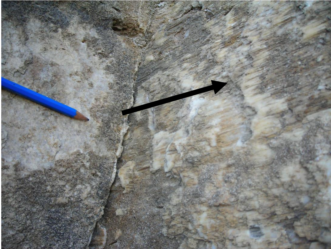
FIGURE 4.6 Fault plane showing dextral strike slip movement as observed from the slickenside lineation.
