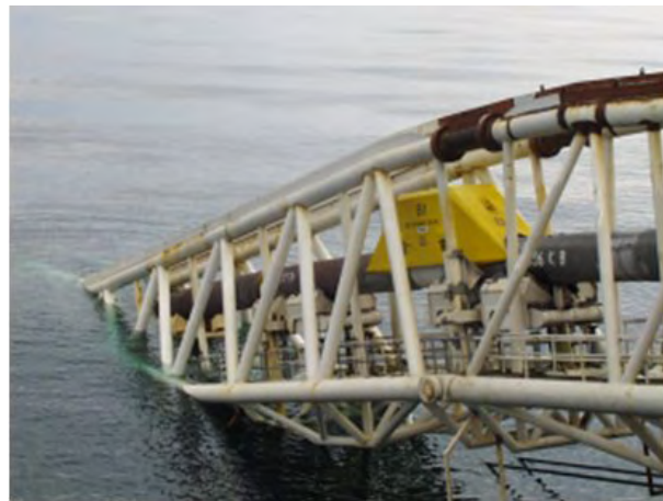
Figure 2.5: Pipeline with HTT over stinger[6].
