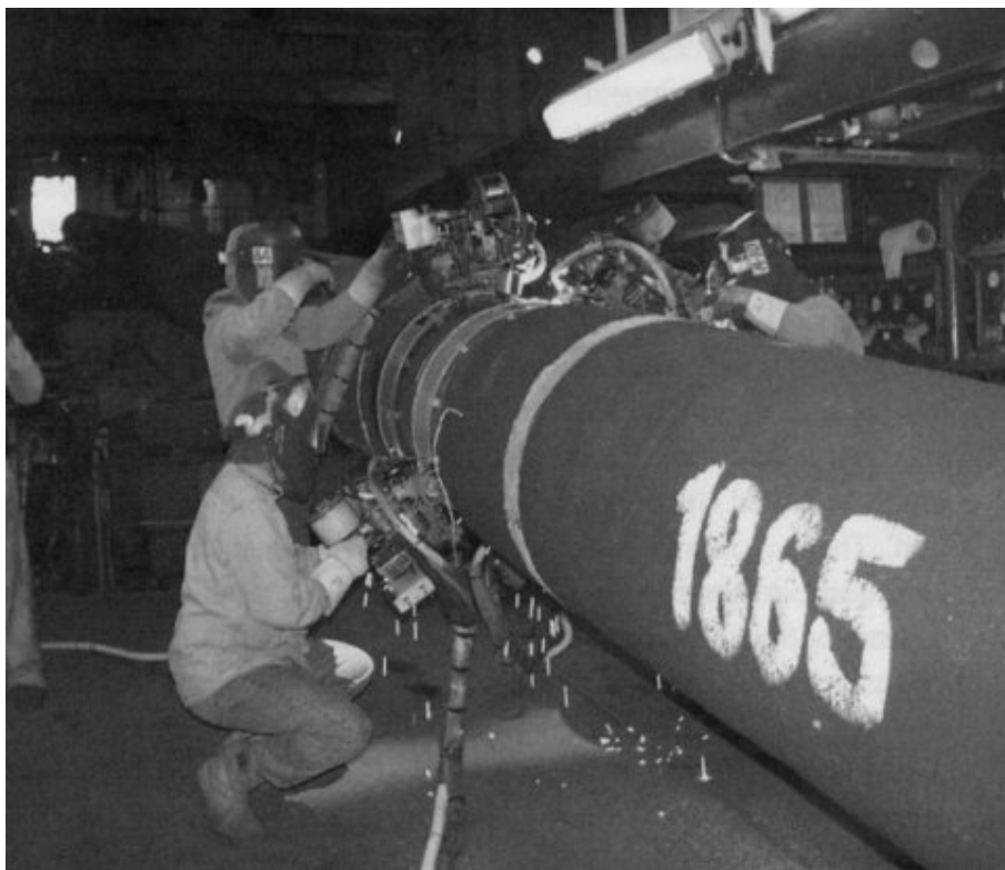
Figure 2.3: Weld station on the lay barge[7]
