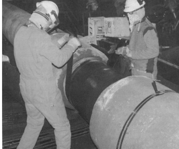
Figure 2.4: Application of field joint coating [7]
