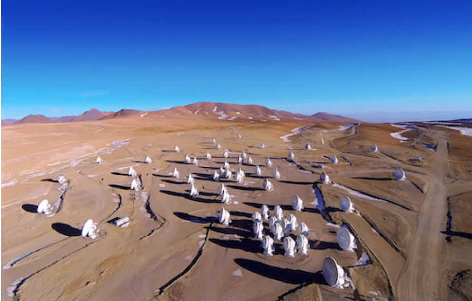
Figure 3.2: This snapshot captures a segment of the ALMA facility. In the centre, you can observe the closely grouped Atacama Compact Array, consisting of twelve 7-meter antennas. They are encircled by four total power antennas and several additional antennas belonging to the main array, which stretches over several kilometres beyond what is visible in the photograph. Image Credit: ALMA (ESO/NAOJ/NRAO)
